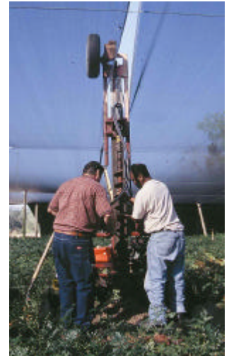
A hollow-stem auger was used to install the multilevel samplers.
