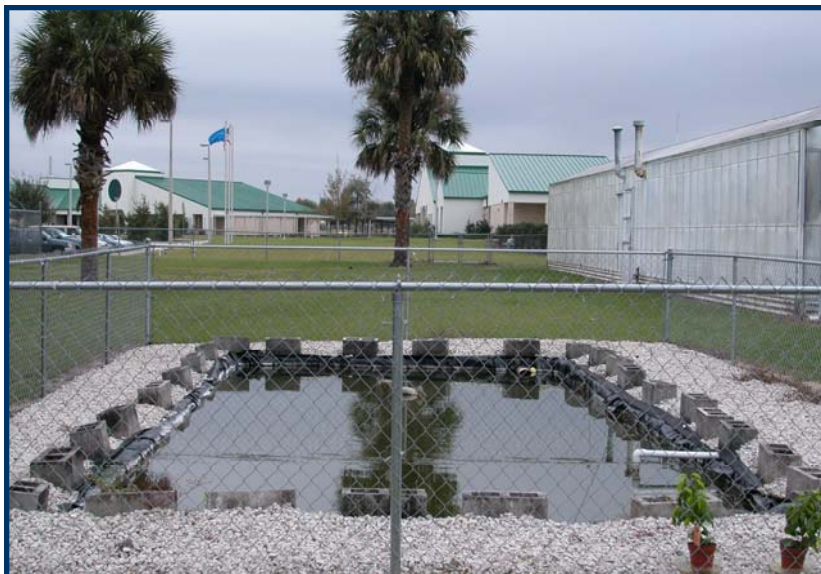
Figure 2. A retention pond capturing irrigation runoff from a production bed and rain water from a greenhouse roof. Water from the retention pond was used to irrigate foliage plants for an entire production cycle.
