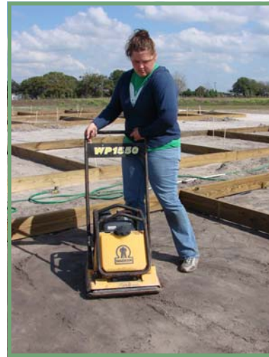
Photo: Compaction of the soil to approximately 1.8 g/cm 3 .
