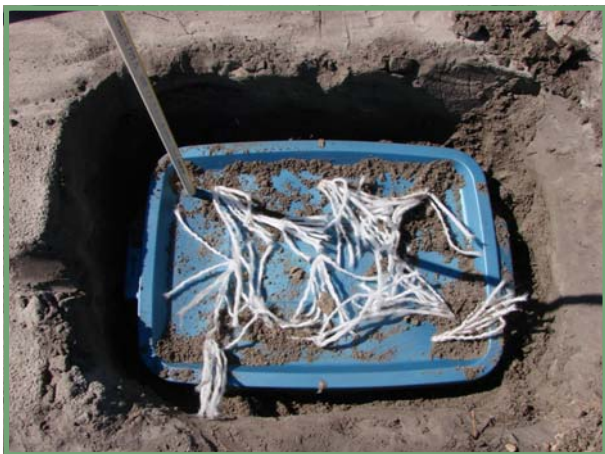
Photo: Installation of leachate collectors
