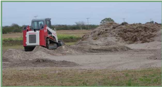
Photo: Removing topsoil and grading the site
